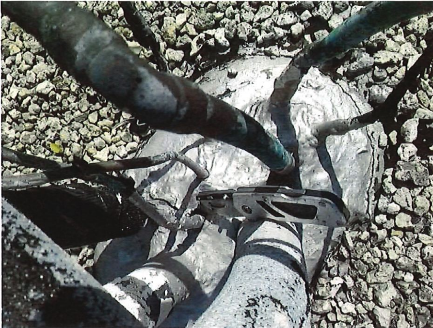
Sealant Deterioration/Failure
